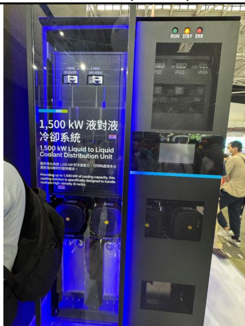
Figure 22: Delta 1,500kW liquid-to-liquid CDU
